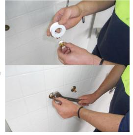
**Step: 4** Centre the Mixermate tap between the 2 pieces of copper tube protruding out of the wall. Mark the copper tube coming out of the mixer tap 10mm back from the centre of the copper coming out of the wall. Cut the copper at these measurements on both pieces of copper. Like before ream out the cut ends of the copper and ensure no filings are left in the tube that may affect the mixer.
