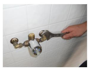
**Step5:** Tighten the elbows onto the mixermate tap's copper tube first so they both face back to the wall. Install the mixer onto position by tightening the other elbow nuts. Have the mixer tap in the off position and turn the water back on. Flush clear any dirty water through another tap before turning on the mixer then flush clear the Mixermate tap before connecting the shower hose. Test for leaks.
