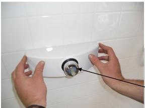
**Step 7:** To install the cover; push the cover over the mixer and back to the wall. Apply silicone to the flat surfaces of the cover to bond securely to the wall. Use a suitable bathroom/wet area silicone.
