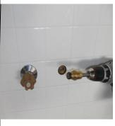
**Step1:** Turn off water supply and remove the old taps. You may need to remove the old tap washers with long nose pliers. Check the condition of the tap seats with a torch. Clean the seat using a Hydroseal re-seating tool to provide a clean finish for the o-ring. Flush out any brass filings to ensure none enter the new mixer. This will void the warranty.
