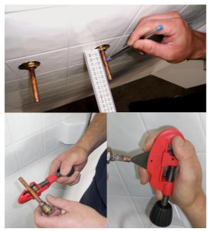
**Step2:** Fit the 2 -piece o-ring and locking nut fitting with the copper tube protruding out of the wall in each tap hole. Measure the copper 30mm off the wall and cut at this measurement on both pieces of copper (that are protruding out of the wall). Ream out the cut ends of the copper and ensure no filings are left that may affect the mixer. (The copper to copper elbows will go onto these pieces in step 5.)
